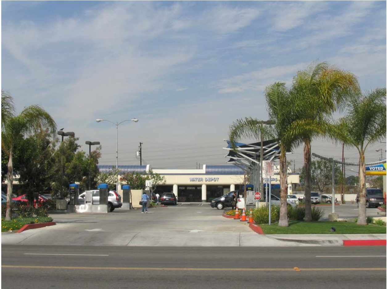
Vacuum Stalls (View from La Palma Ave)
