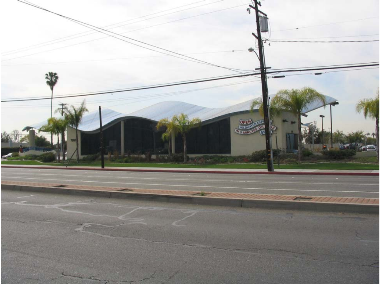
Wide Angle View of Eastern Elevation (Facing Knott Ave)
